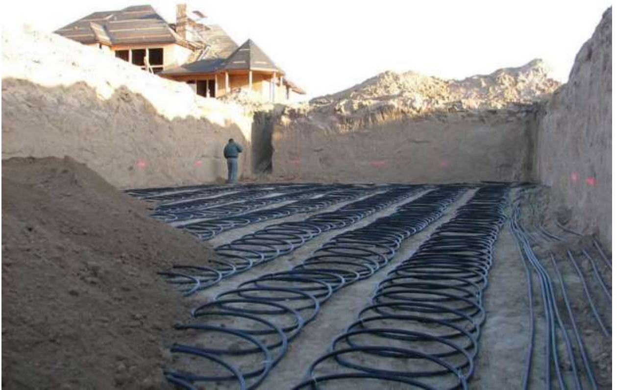
(1-rasm. Gorizontal geotermal issiqlik nasosi )
