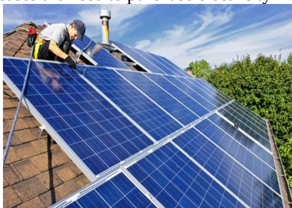
Figure 1. Rooftop solar panels installation
